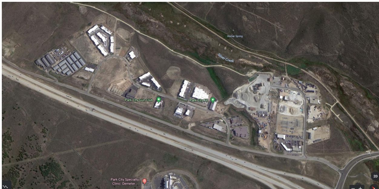
Figure 1 Aerial View of the Service Commercial Zone
